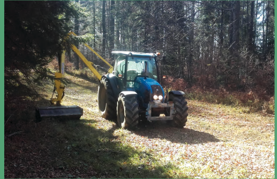
Mulching of slopes of forest roads and overgrowing forest clearings
