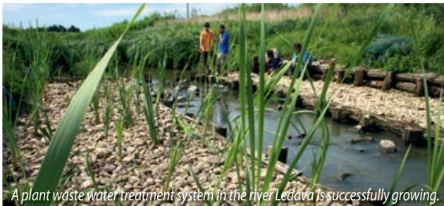
Indentation forming, using wooden piles
