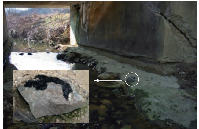
Newly constructed shelf under the bridge was immediately accepted and marked by the otters.
