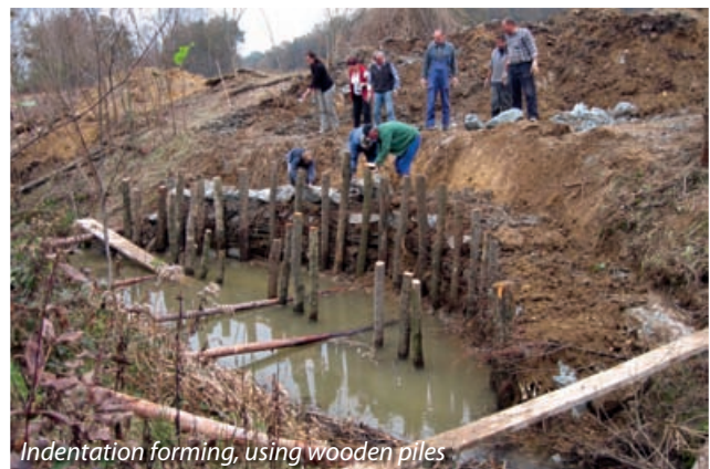
Putting the wooden nail into the riverbed
