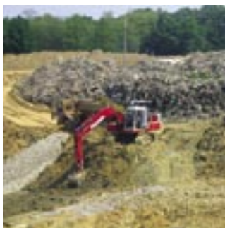
↑ Izkop starih odpadkov in onesnaženih zemljin Excavation of old wastes and contaminated soils
